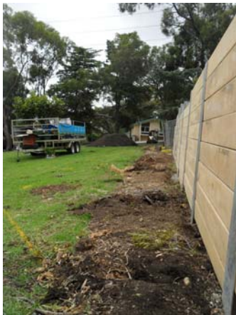
1. Digging up grass to prepare the area for planting
